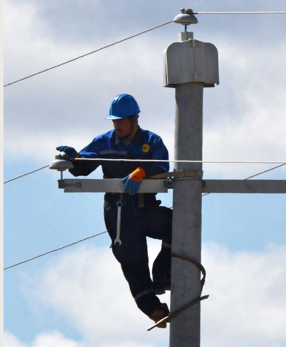
Mongolian utility company engineer insulating a power pole. (Photo by Munir Virani - MBZRCF)
