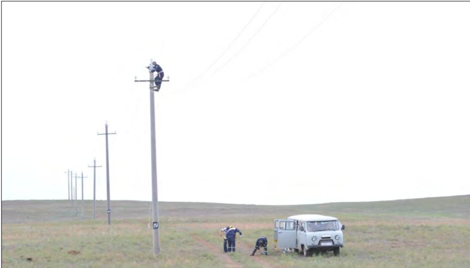
(Above): Mitigation work undertaken on a dangerous power line in Mongolia
