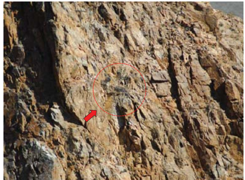
6. N06 on the inaccessible cliff
